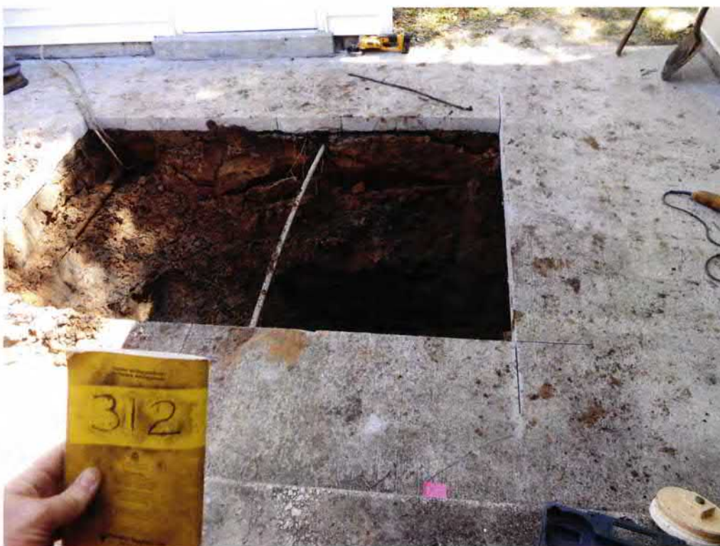
Picture 2: UST 312Ash excavation.
